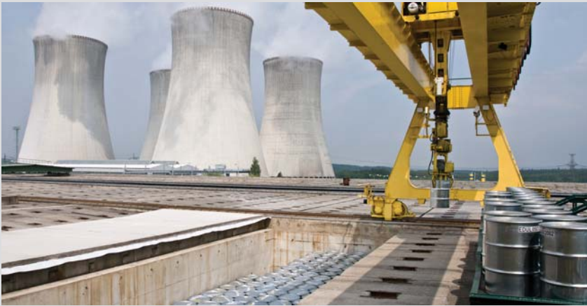
The Dukovany repository consists of 112 reinforced concrete vaults arranged in four rows of 28 vaults each.
