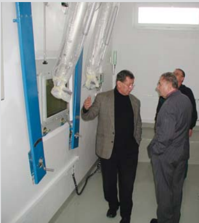
An inspection day during the refurbishment of the hot cell at the Richard repository.
