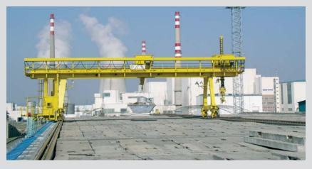
The repository consists of 112 reinforced concrete vaults arranged in four rows of 28 vaults each. The waste drums are placed within the vaults by a gantry crane; the operator's cabin is shielded to protect the operator from radiation exposure.
