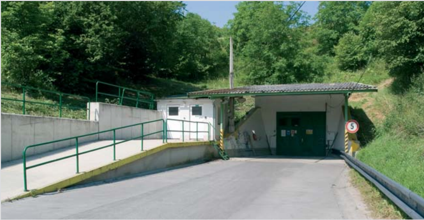
Entrance portal of the Richard repository.
