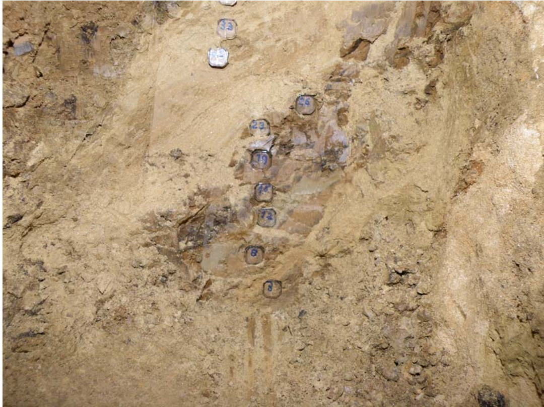
Photo 2 Segment HH03 to HH33
