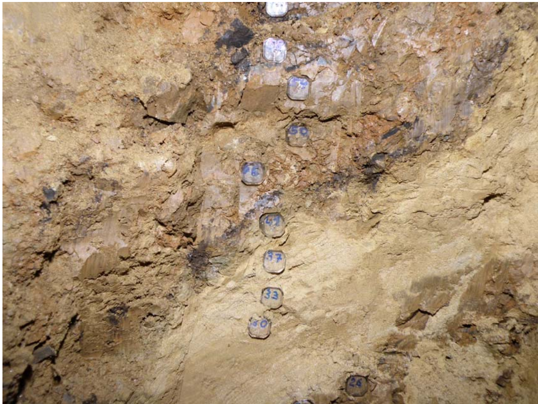
Photo 3 Segment HH26 to HH58
