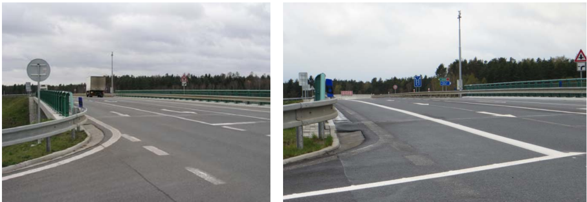
Fig. 2 Left turn sight before and after the change of road marking (source: CDV and ŘSD)
