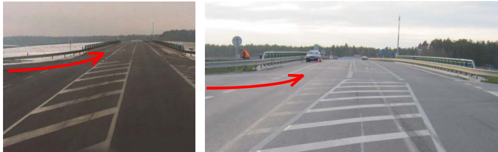
Fig. 2 Left turn sight before and after the change of road marking (source: CDV and ŘSD)
