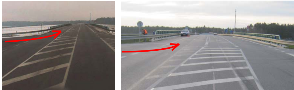
Fig. 2 Left turn sight before and after the change of road marking (source: CDV and ŘSD)
